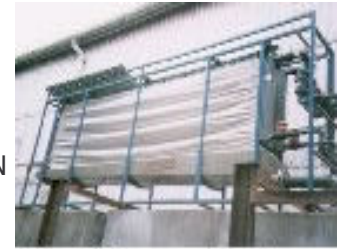
Liquid by-product recovery and re-use using membranes
